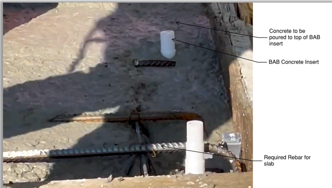
Figure 3: Concrete being poured around BAB inserts
