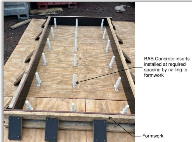
Figure 1: BAB Concrete insert installation demonstration
